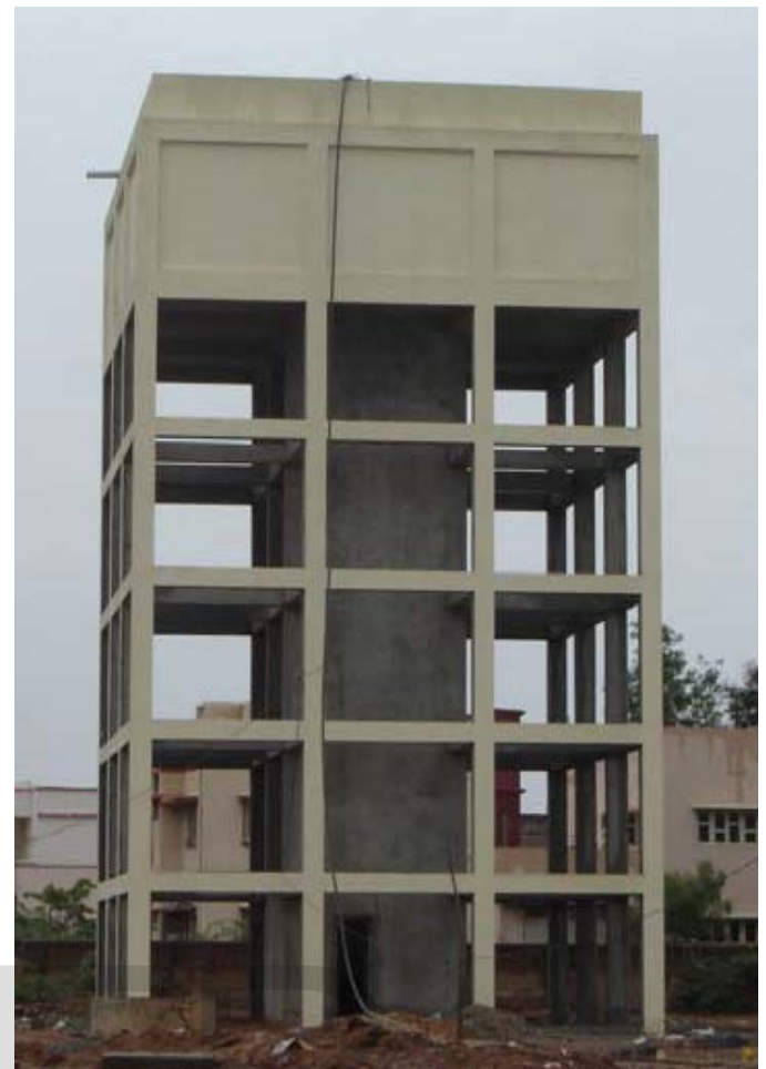
Fig -1: Existing water tank at Bhuj
